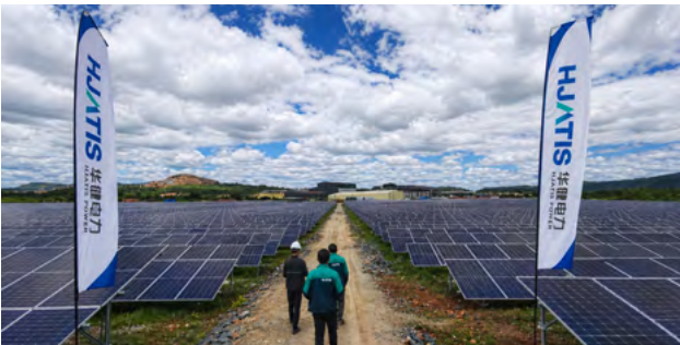
Almid Smelter Centralized PV Plant
