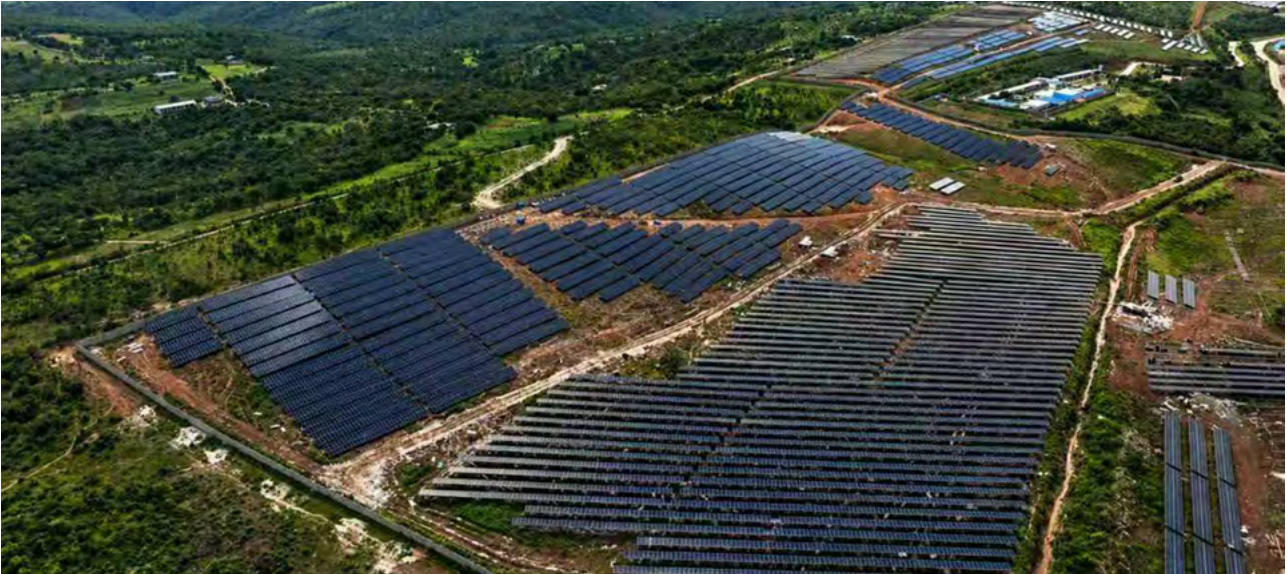
CNBM Industrial Park Green Energy Supply
