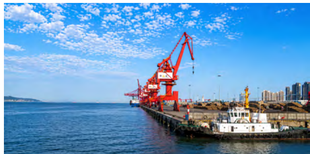
GBG Bauxite Port Phase I Project
